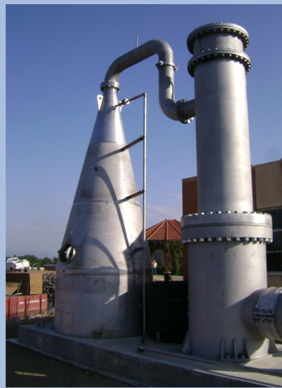
Installation of ECO 2 's Speece Cone in Marston Reservoir
