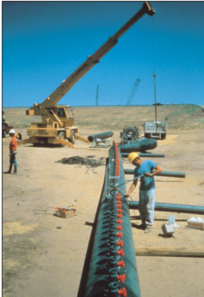
View of the 150-foot long diffuser used to distribute oxygen-rich water in the hypolimnion layer of the lake.
